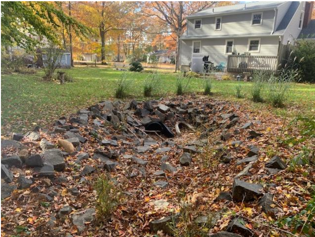
Photo 5: Receiving Culverts behind 113 Blatchley Ave
