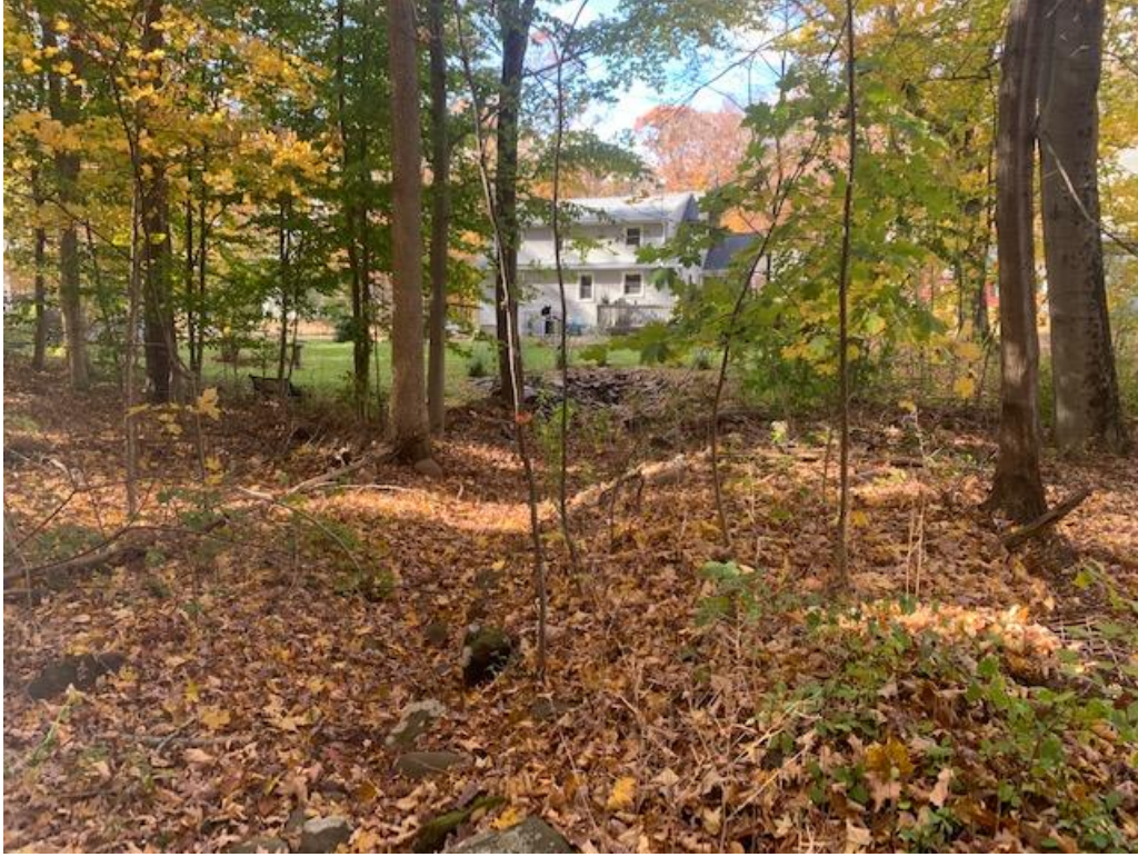
Photo 4: "flow" path heading towards receiving twin culverts behind 113 Blatchley Ave
